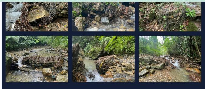
DAMAGE. Soil erosion mitigation of Petrowind faces setbacks, with damaged gabions along the Napaan River. Photo courtesy of Malay LGU engineering department
